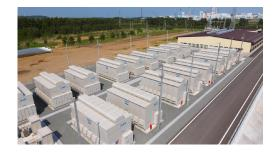
NaS technology: promising battery technology for grid scale storage. Hot temperature operation (300°C). Deals with Terna (Italy) and EDF (France).
